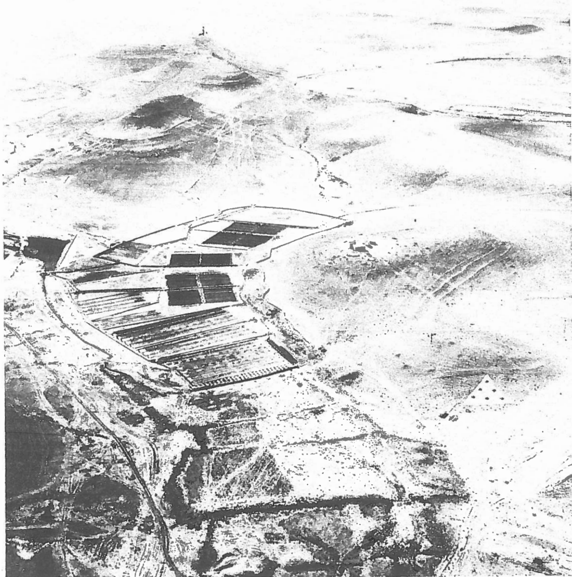
Fig. 111. Aerial photograph of the Avdat farm. In the foreground are four unreconstructed terraces of the ancient farm. The farmhouse is on the hill at the right. Blocks 1-14 can be easily identified (compare Fig. 113). In the background are six reconstructed channels leading runoff from the hills to the various weirs. On the hill to the right of the farmhouse the traces of three unreconstructed channels can be seen. In the background are remains of ancient farms.
